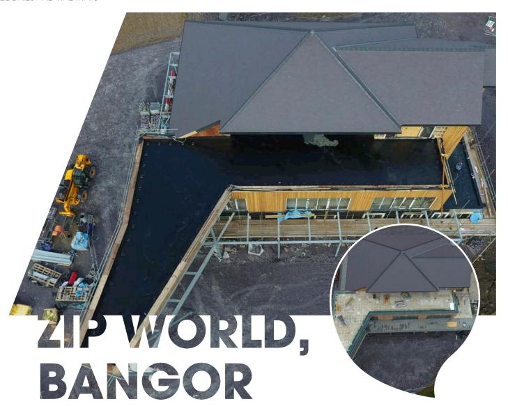
Proteus Waterproofing systems provide fast and efficient installation for long term, all-weather protection as can be seen below with the new build terrace roof project at Zip World, Bangor.
