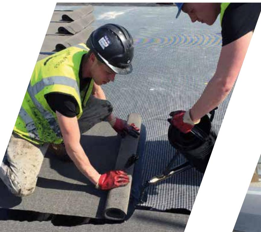
The Hot Melt waterproofing compound has been engineered as a buried structural waterproofing membrane and forms the waterproofing to the Proteus Hot Melt® system, incorporating insulation and finishes for inverted roofs such as green or ballasted roofs.
