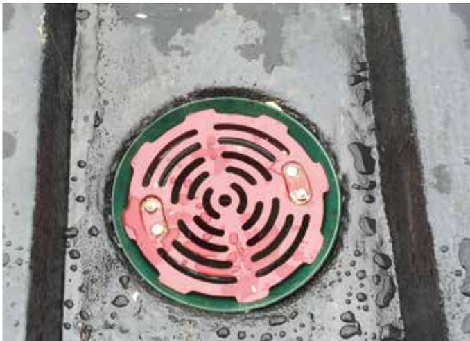
Install a rainwater outlet of the required diameter prior to installation of the **Cold Melt**<sup>®</sup> membrane. Apply **Pro-Prime**<sup>®</sup> SA first, followed by **Pro-Carrier Membrane SA**, to the primed concrete surface ensuring a full bond. Dress the **Pro-Carrier Membrane SA** onto the membrane flange a minimum of 100mm. Please note; a slight water check could be created when dressing onto the membrane flange.
